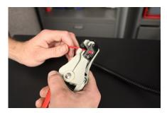
**B.** Place wire from add-a-fuse and WH-1006-3 into butt connector. Using crimping tool connect add-a-circuit and WH-1006-3 with butt connector. Install appropriate fuse into bottom slot (opening that is near the spade).
