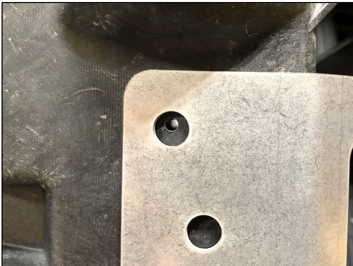
FIGURE 23 : Pre-Drill Hole Position
