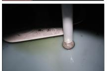
N. Install Bulkhead with lock washer and nut. Tighten nut securely with a 1-7/8" socket or wrench. Make sure the fittings are unobstructed.
