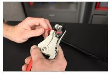
B. Place wire from 46044 and WE-1001 into butt connector. Using crimping tool connect 46044 and WE-1001 with butt connector. Install 46260 to 46044 bottom slot (opening that is near the spade). Route 46044 lead through the fire wall using existing grommet.
