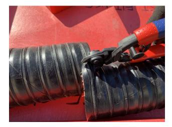
Install End Cuffs (V, *HP1359-00*) and #56 Hose Clamps (G, *HP1359-00*) onto both ends of the Flexible Duct (E).
