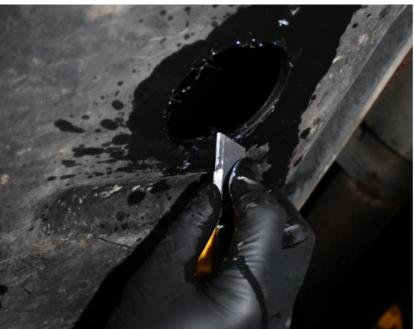
3. Thoroughly de-burr the edges of the hole and remove any high spots on the outside of the tank using a razor blade.
